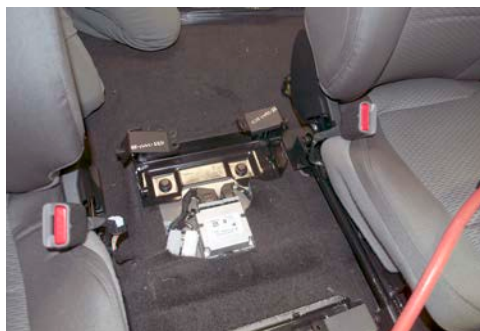
Loosely mount Floor Plate Feet, as marked on feet for location, onto sides of OEM brackets re-using (4) OEM 1/2" bolts.
