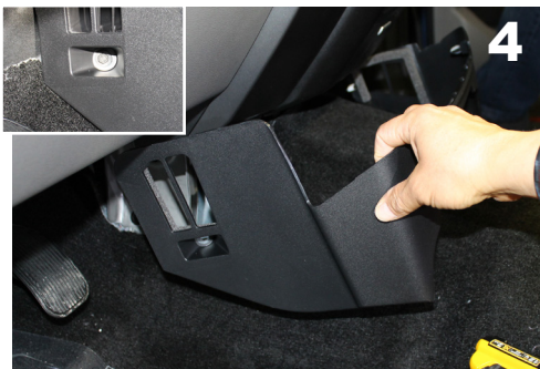
Remove (1) 10mm screw holding the lower trim in place rotate over the transmission hump and unsnap from the passenger side.
