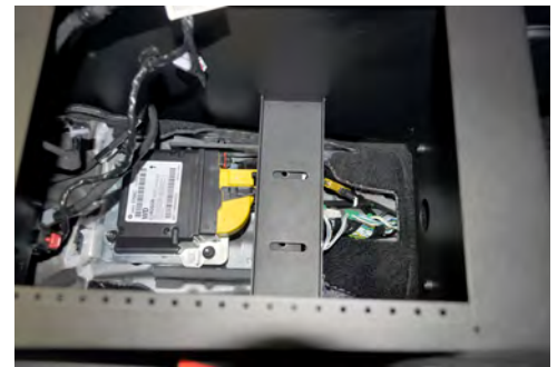
Reroute all OEM wires and reconnect.
